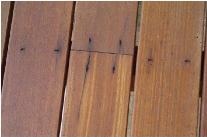
Photograph 3 - Iron staining due to ungalvanized nails (also nails are not appropriate type)
