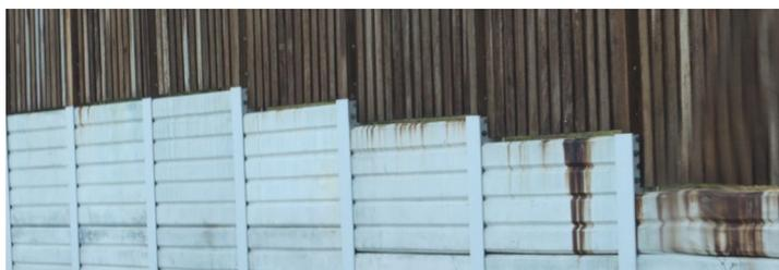
**Photograph 1 - Unpainted hardwood causing tannin stains on concrete**
